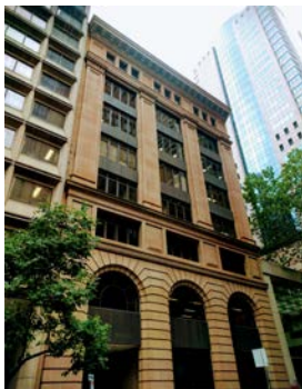
LSC's new accommodation
